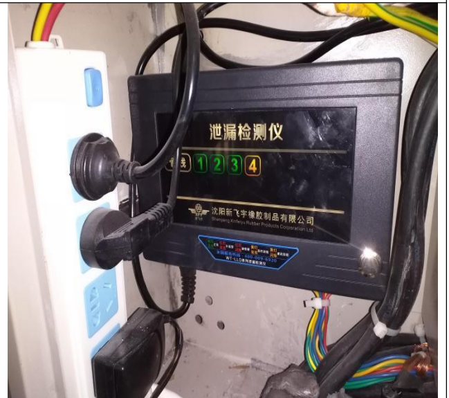
输油管线渗漏检测
